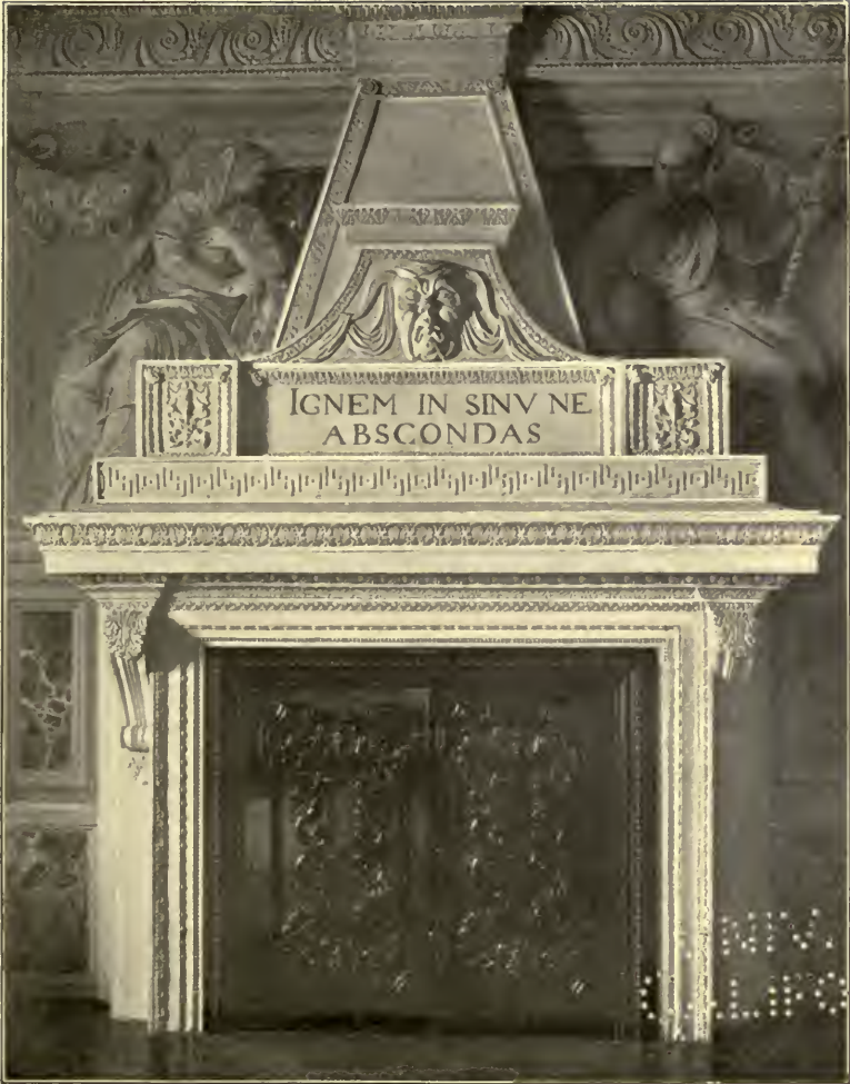
MANTELPICE IN THE VILLA GIACOMELLI, AT MASER. NEAR TREVISO. XVI CENTURY. (SHOWING IRON DOORS IN OPENING.)
